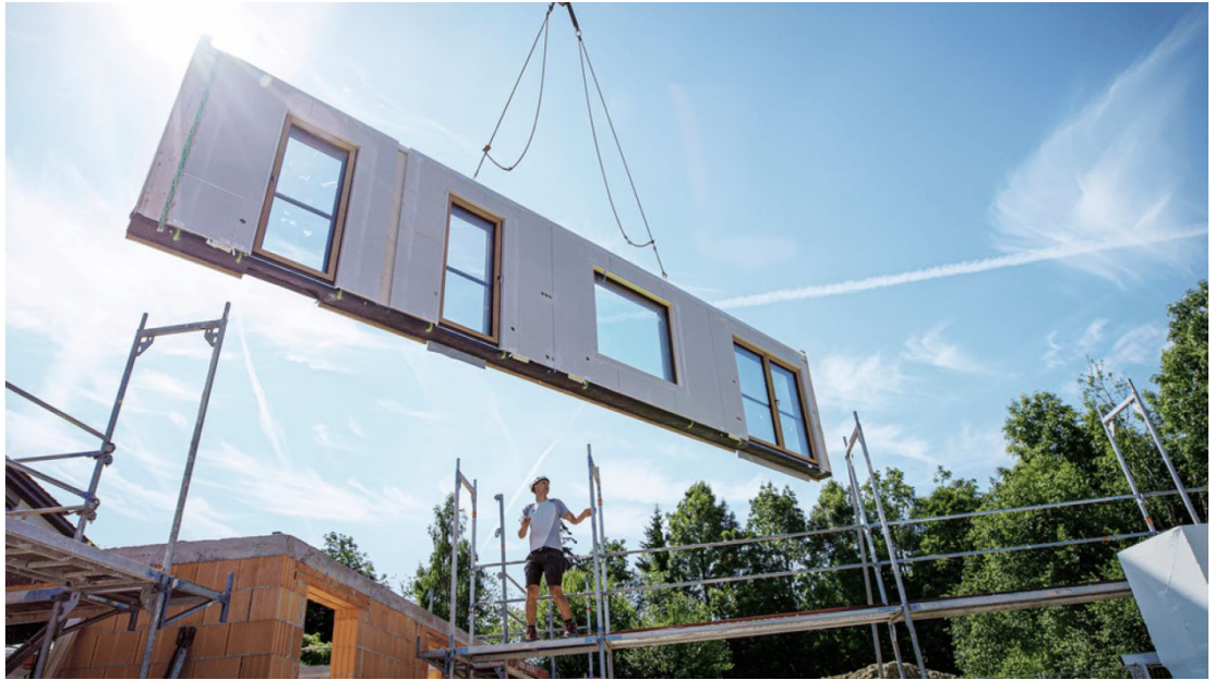
Fig. 2.5: Installation of a prefabricated timber panel on site
