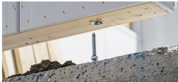
Fig. 2.6: Positioning of the HCW on top of the post-installed anchor with a levelling nut
