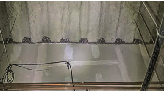
Fig. 26: Hilti CFS-TTS MD installed correctly per EJ
