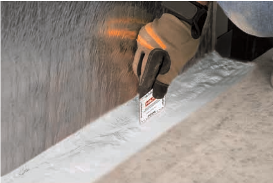
Fig. 33: Correct depth of sealant, Hilti CFS-SP SIL
