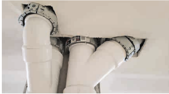
Fig. 15: Multiple cable collars Hilti CP-643 N used for sealing a large opening, leaving gaps in the installation
