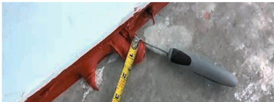
Fig. 7: Sealant thickness measurement when wet
