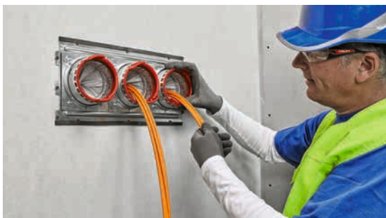
Fig. 10: Speed sleeve with gang plate, Hilti CFS-SL GA used for small cable bundles
