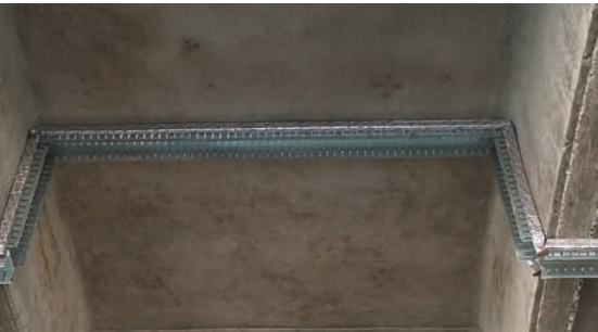
Fig. 25: Hilti CFS-TTS used on top of wall joint
