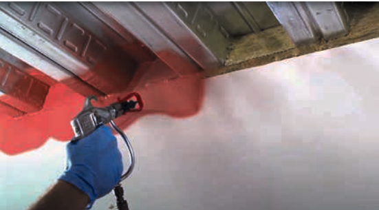
Fig. 28: Hilti CFS-TTS MD installed correctly per EJ
