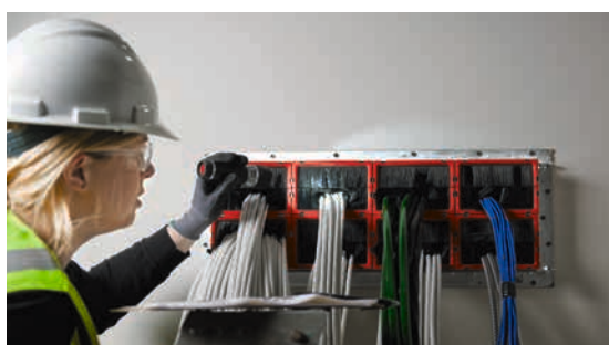
Fig. 11: Group of modular sleeves with gang plate for sealing multiple cable bundles of different sizes Hilti CFS-MSL GPA. Watch the video
