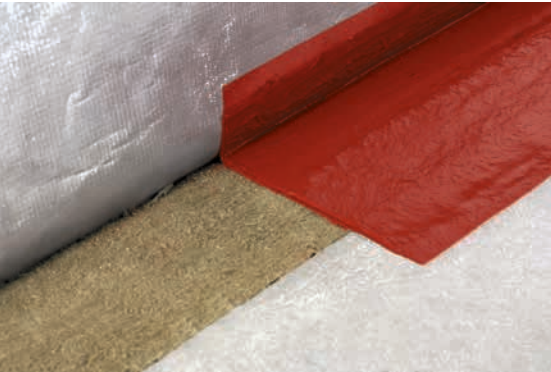
Fig. 32: Sealant Hilti CP-672, application in edge of slab assembly
