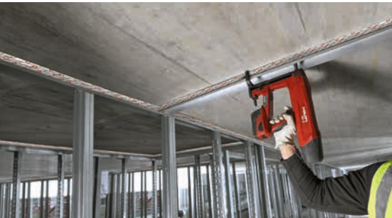
Fig. 24: Hilti CFS-TTS used on top of wall joint Watch the video
