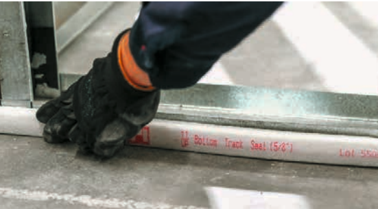
Fig. 27: Bottom track seal installed on floor runner
