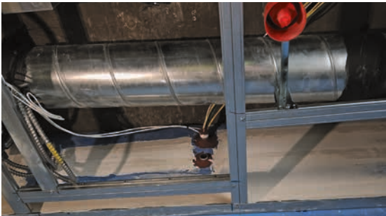
Fig. 16: Blank opening (bottom one out of two sealed small openings)
