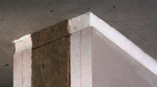
Fig. 22: Flexible firestop sealant (Hilti CP606 - white) applied to both sides of the wall with mineral wool backing material
