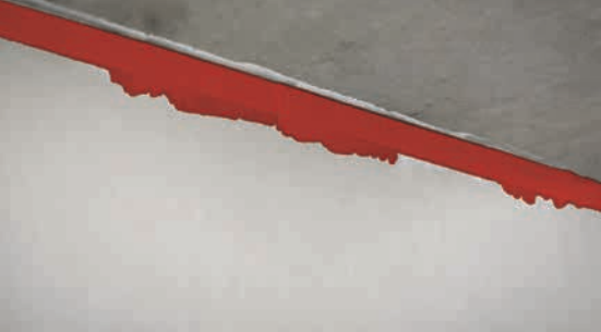
Fig. 23: Firestop sealant applied to the top-of-wall joint
