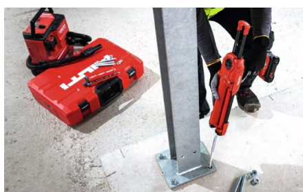
a) Adhesive mortar injection
