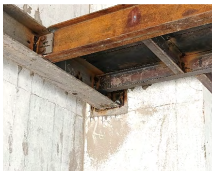
b) Post-anchoring application for baseplate connection
