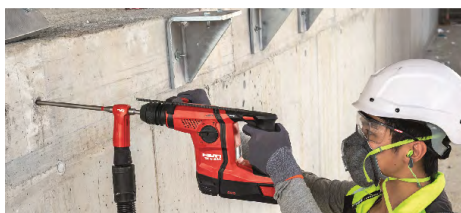
b) Drilling being done for horizontal application
