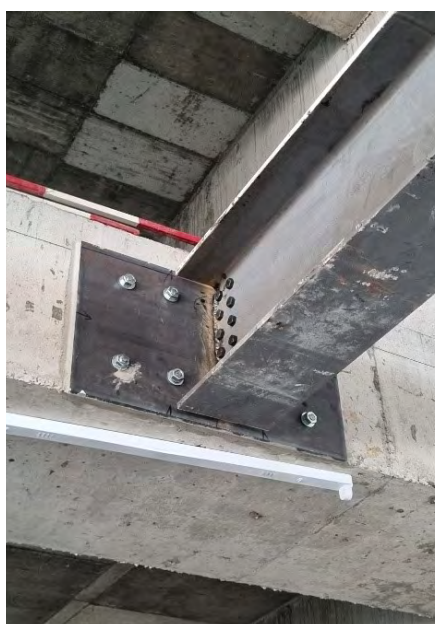
c) Detail of steel to concrete connection
