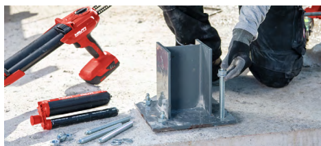
a) Anchors installed in vertically downward direction
