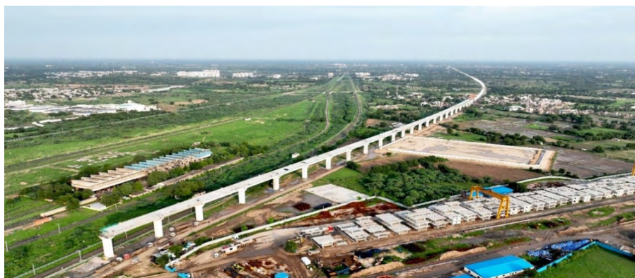
a) MAHSR viaduct portion
