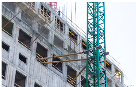
b) Tower crane support
