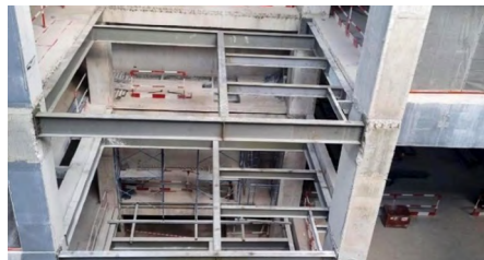
b) The steel frames are connected by anchors to the reinforced concrete structure
