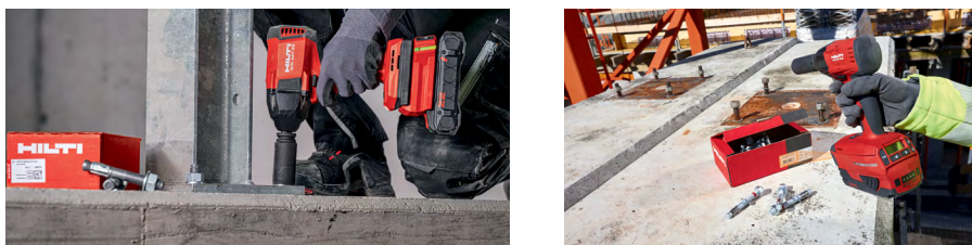
Fig. 8.16: SIW system torque wrench and AT module
