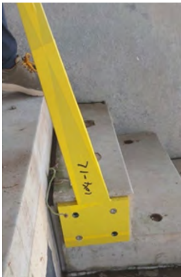
a) Baseplate application during construction
