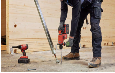
a) Drilling holes with a Rotary hammer
