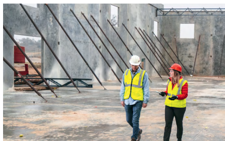
a) Temporary wall support
