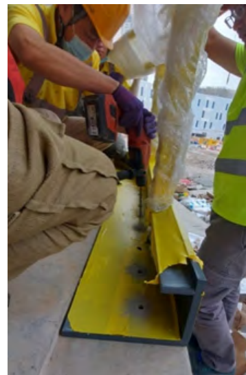
c) Placement of steel profile
