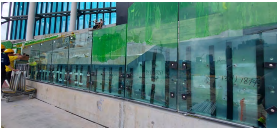
a) The structure at job site
