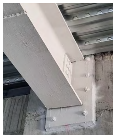
Fig. 6.11: Baseplate connection using group of anchors (4x2)
