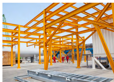
a) Primary steel column
