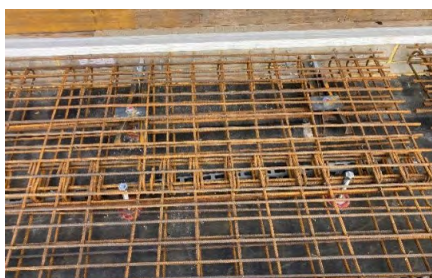
b) Anchors in rebar before pouring concrete
