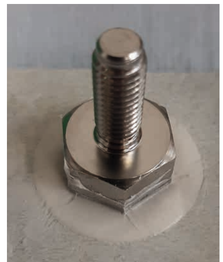
Repaired opening of PFP-coating
