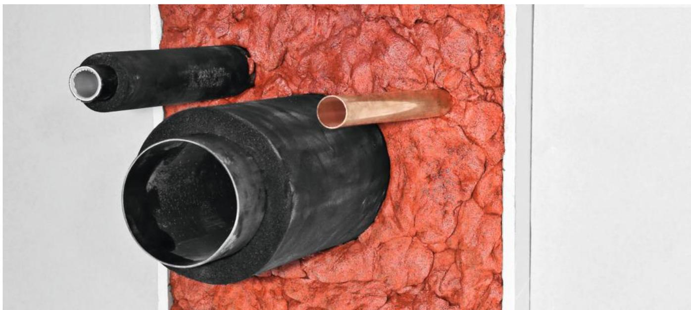
**3.1 ATTRAVERSAMENTO DI TUBAZIONI METALLICHE COINBENTATE IN APERTURE DI DIMENSIONI MASSIME 400 X 400, CON SCHIUMA HILTI CFS-F FX (ETA 10/0109)**
