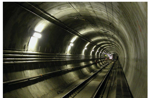
Figure 5: Civil Construction (pre-cast)
