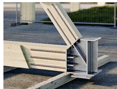
b) Timber-to-steel plate
