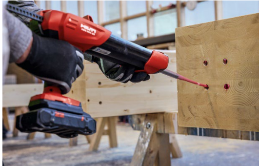
Fig. 2.5: Hilti GiR installation with direct filling
