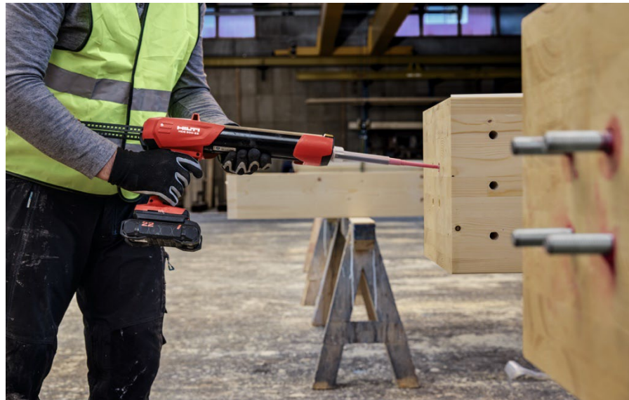
Fig. 2.1: Hilti HIT-RE 500 V4 glued-in rods
