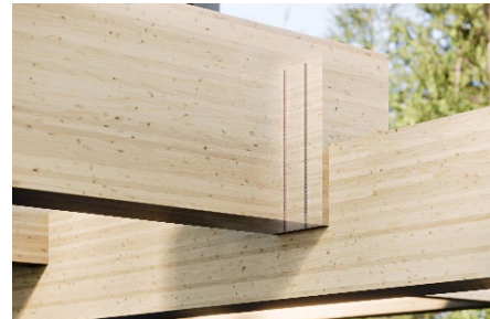
b) Notched reinforcement
