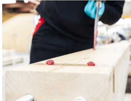
Fig. 2.3: Hilti GiR installation with bypass filing
