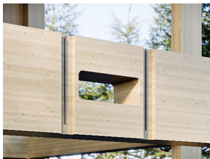
c) Holes in beams
