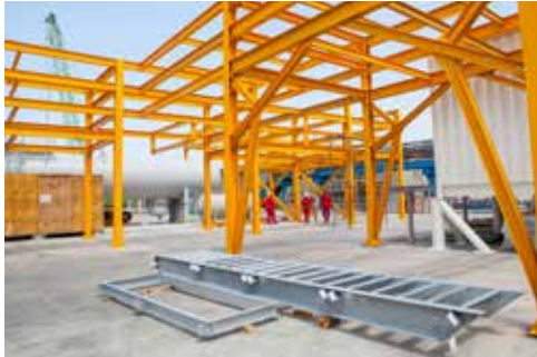
Primary steel column
