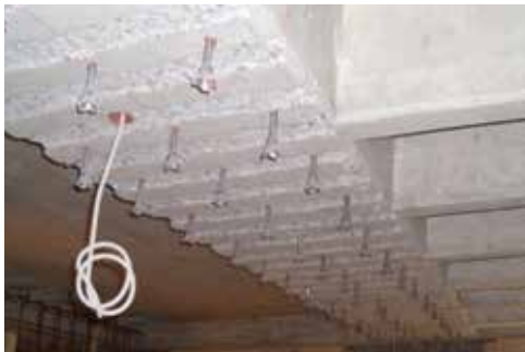
Increasing RC beam depth
