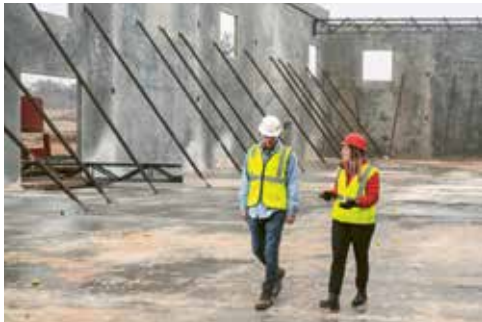
Temporary wall support
