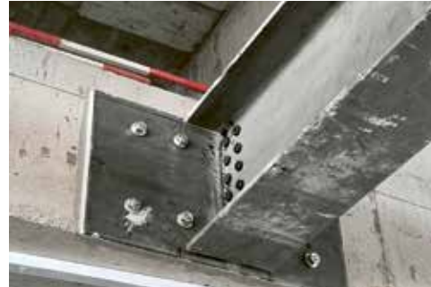
Primary steel beam
