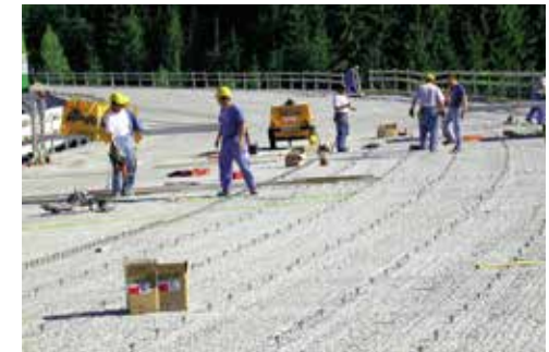
Increasing bridge deck slab thickness
