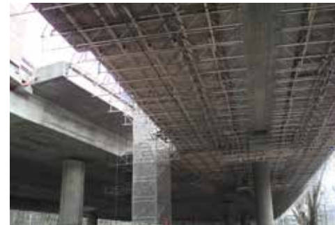
Increasing bridge girder thickness
