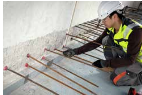
Slab-to-wall connection
