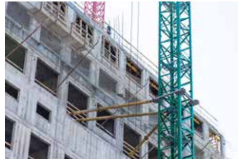
Tower crane support
