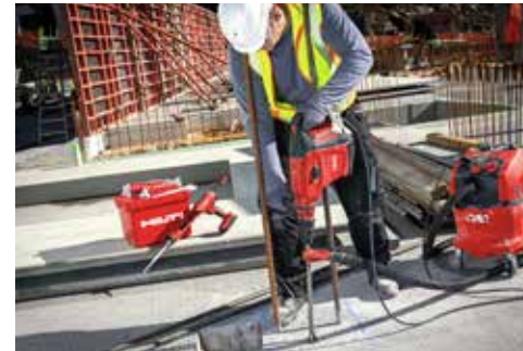
Column-to-slab connection
