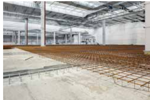
Strengthening of industrial floor
