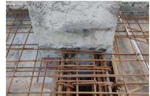
Beam-to-column connection
