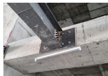
b) Steel beam-to-concrete connection
