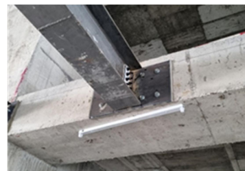
b) Steel beam-to-concrete connection
