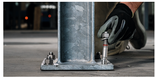
b) Steel-to-concrete connection
