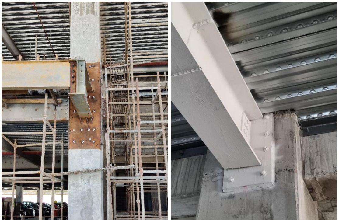
Fig. 1.1: Critical anchor arrangements at jobsite
