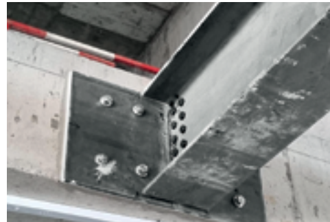
Primary steel beam
