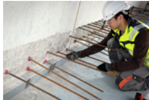
Slab-to-wall connection
