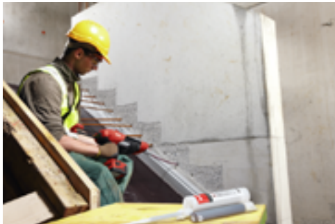
Stair-to-wall connection
