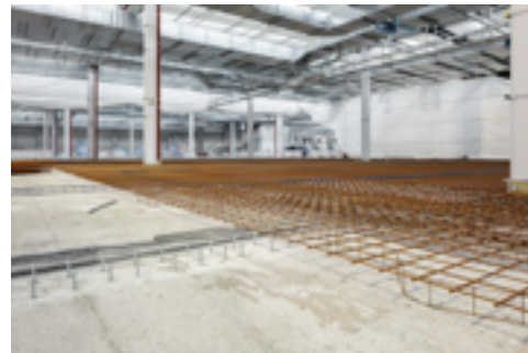
Strengthening of industrial floor
