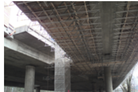
Increasing bridge girder thickness
