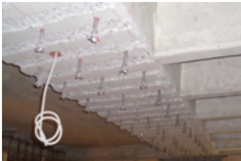
Increasing RC beam depth
