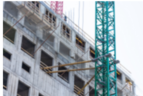
Tower crane support
