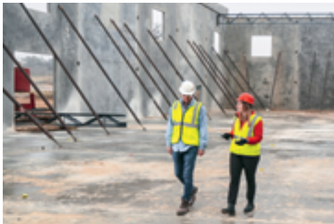
Temporary wall support
