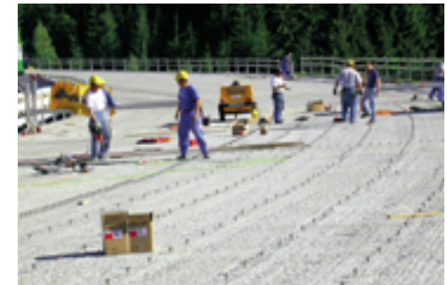
Increasing bridge deck slab thickness
