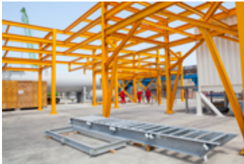
Primary steel column
